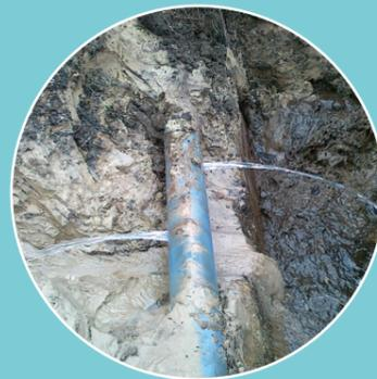
Leaks on pipe in rural area. Serious leakage of 400,000 m<sup>3</sup>/y. It did not surface but was found when sectioning the network and by manual leak detection.
