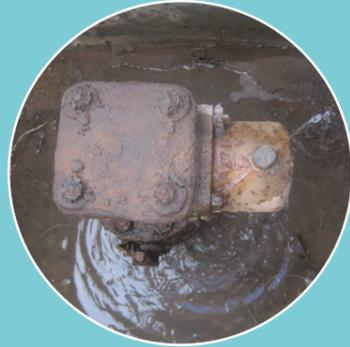
Leaking valve in valve chamber. Leaking 500 m<sup>3</sup>/y. Regular valve surveys would minimize the run time of such leaks.
