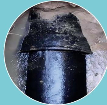
Buried leak that does not surface. Leaking 2,500 m<sup>3</sup>/y. Active leakage control would lead to shorter run time.
