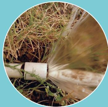
Temporary above-ground installation that has become permanent. It leaks around 3,500 m<sup>3</sup>/year.
