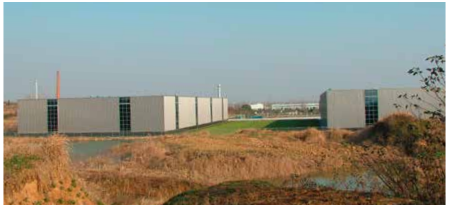
The new machining factory building (at left) is built next to the existing fitting factory buildings (at right).
