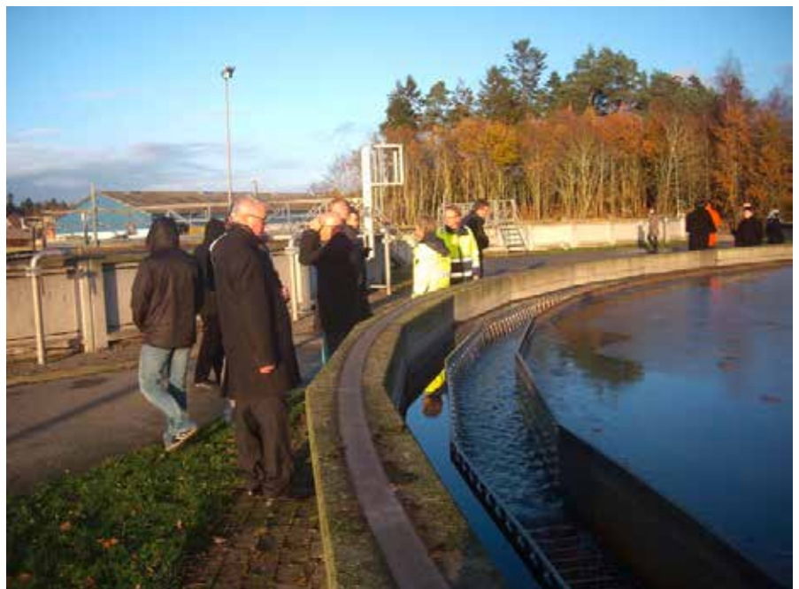
Skanderborg wastewater treatment plant.
