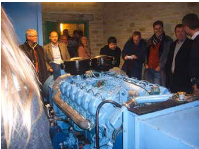
Horsens Vand A/S, Rugballe Waterworks - diesel generator.
